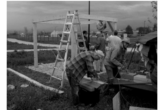
Eyeopener's construct a shelter on the Mason Street Trail
